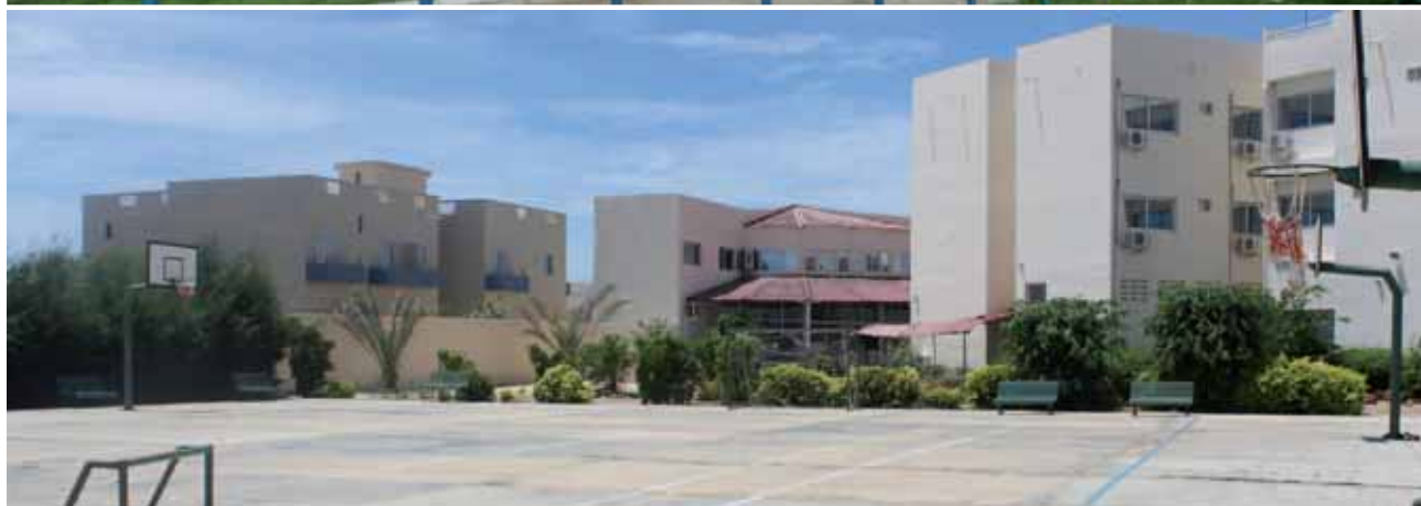
Top: The new AfricaRice Regional Training Center, Boudiouck, Saint-Louis, Senegal. Bottom: Dedicated recreation area for trainees' and trainers' use at the new Regional Training Center
