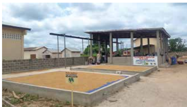
Traditional rice drying (left: Goronyo, Nigeria) and improved rice drying surface (right: Glazoué innovation platform, Benin). The clean concrete surface and surrounding walls of the improved infrastructure protect the drying rice from a high proportion of the impurities that laying the tarpaulin on the ground exposes rice to in traditional drying.
